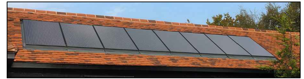
In tile PV solar panels on south face of roof
